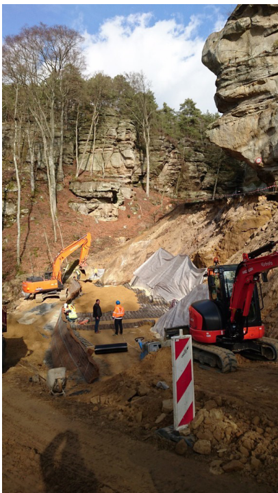
Figure 11: Stabilisation system under construction.
