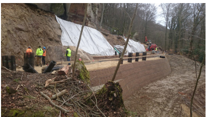
Figure 12: Rock outcrop integrated into the stabilisation system.
