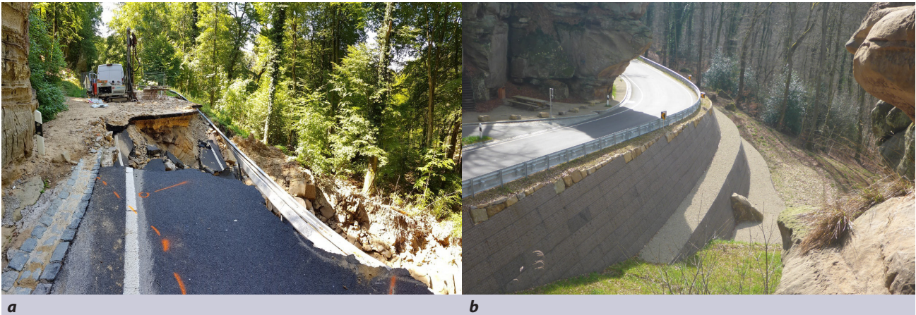
Figure 13: Situation before (a) and after (b) stabilisation.
